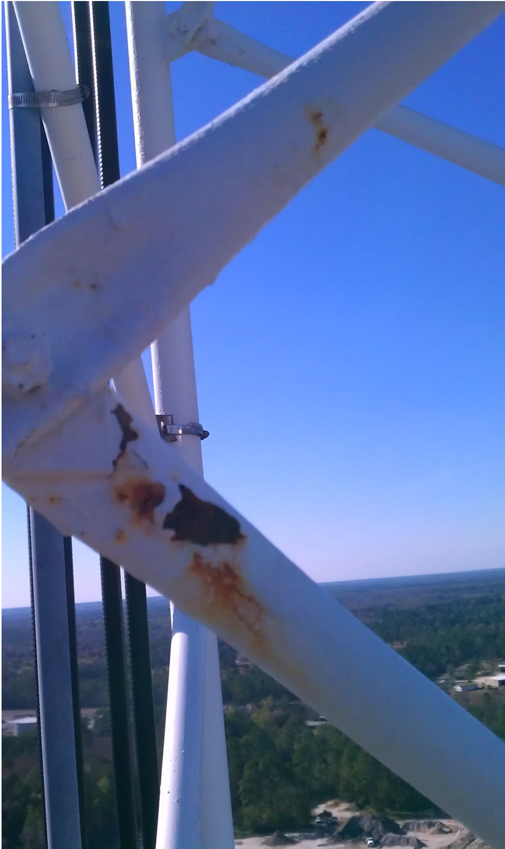
3. At Approximately 340 Feet.
