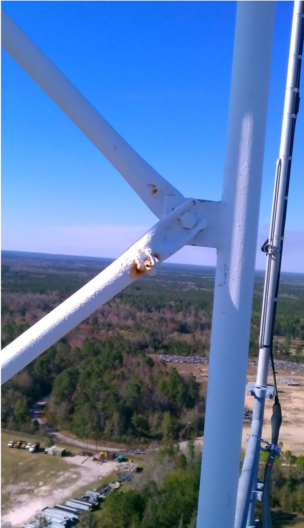
1. At Approximately 340 Feet.
