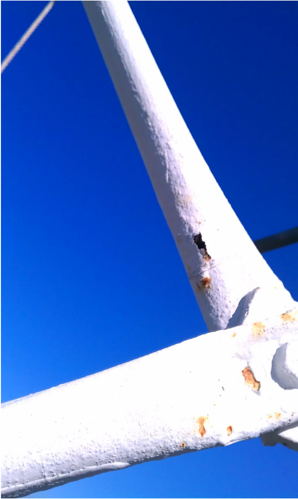
2. At Approximately 340 Feet.
